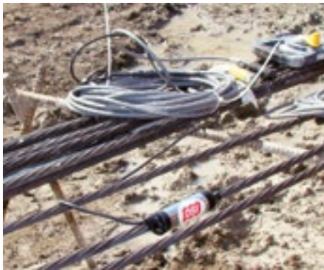
DYNA Force® for force monitoring of tie-back anchors at Park Place, Toronto, Canada
