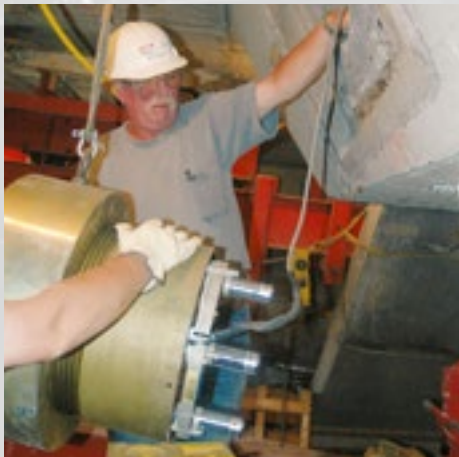
DYNA Force® in Cable Stay Anchorage, Penobscot Narrows Bridge, Maine, USA
