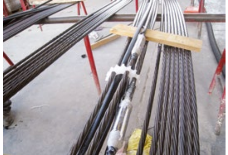
Installation of DYNA Force® Sensor over strand anchor bond length
