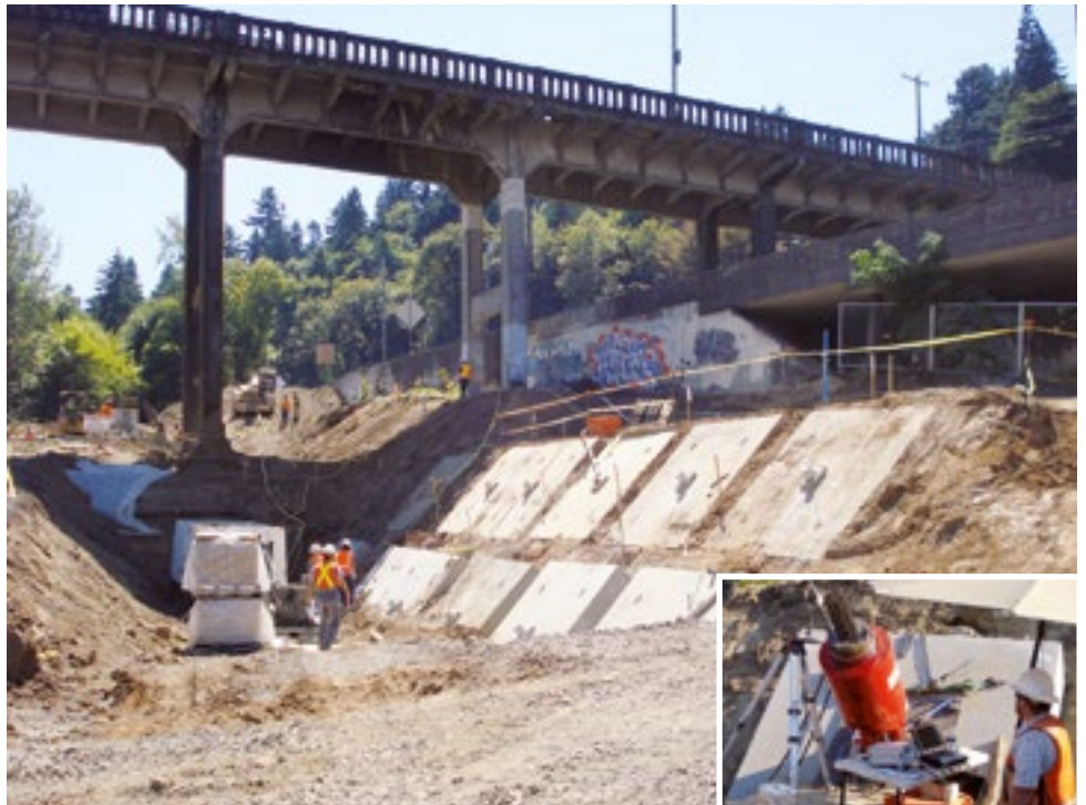
DYNA Force® for ground anchors at Sellwood Bridge, Oregon, USA
