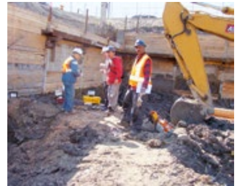
DYNA Force® for force monitoring of tie-back anchors at Park Place, Toronto, Canada
